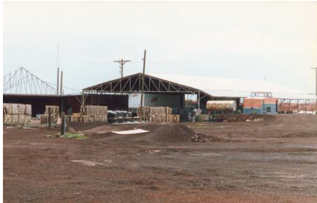
Flower rock packing plant and diesel mechanical loco.
