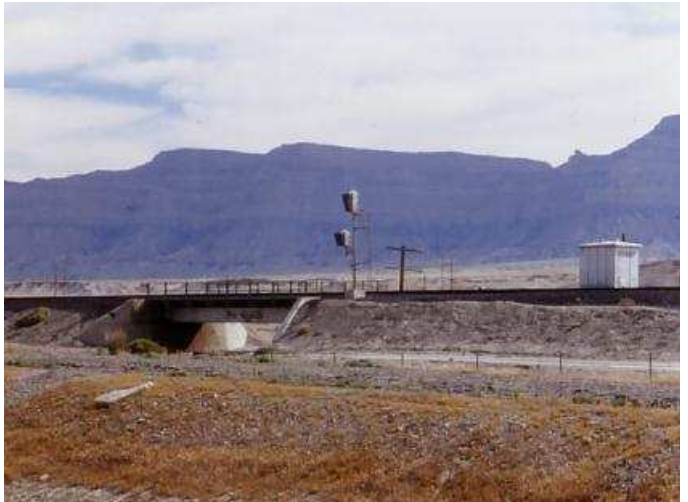
Above; Structures at the western end of the siding at Desert.
